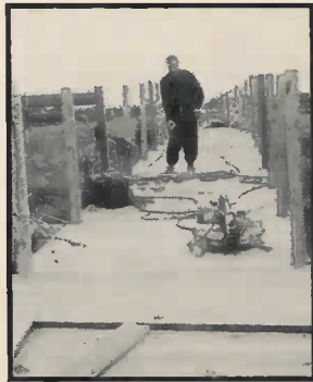
Working on the Boardwalk
